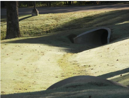
Figure 16.2 (above) Underground drainage piping with grassed swales provides a more aesthetic and environmentally friendly solution rather than the rip-rap swale in Figure 16.3 (below) .
