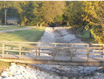
Figure 16.2 (above) Underground drainage piping with grassed swales provides a more aesthetic and environmentally friendly solution rather than the rip-rap swale in Figure 16.3 (below) .
