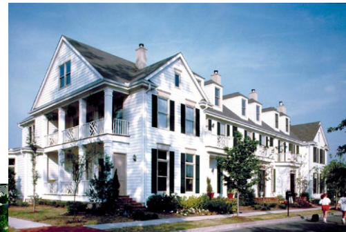
Figure 8.3 (left) Well planned residential neighborhoods, such as Harbor Town, create well defined and organized thoroughfares with easy access to points of interest. Greenspace is easily accessible and has been incorporated into the design purposefully.
