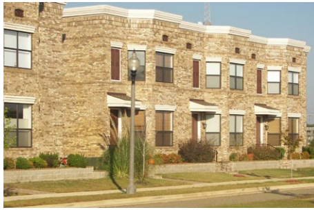
Figure 8.2 (below) This multi-family building is inviting with close interaction to the street and sidewalk.
