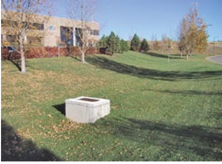
Figure 16.1 Stormwater detention areas like this one are used to slow excess stormwater runoff from the site without proving to be an eyesore.
