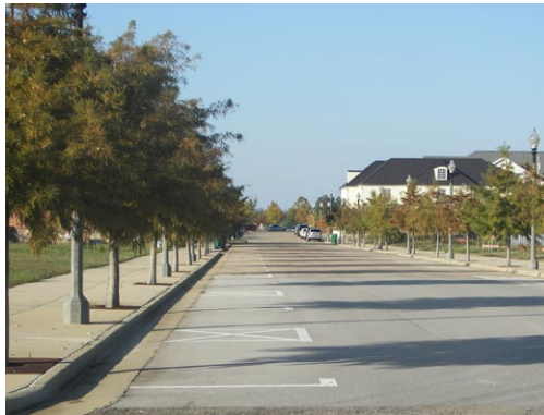
Figure 10.2 Street elements such as on street parking, decorative street lamps and tree islands promote an urban street environment.
